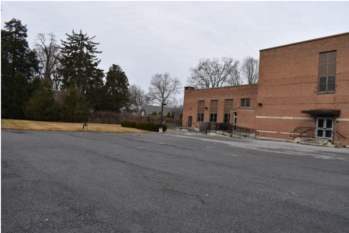
Photo 2: The southern portion of the Parcel contains an asphalt covered parking lot. View to the northwest.
