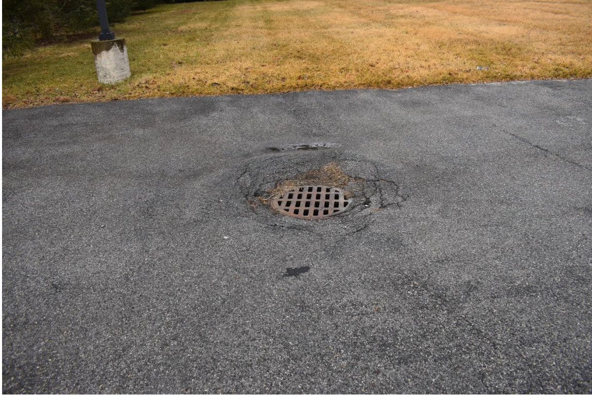
Photo 13: Stormwater drains are located in the parking area, in the southern portion of the Parcel. View to the west.
