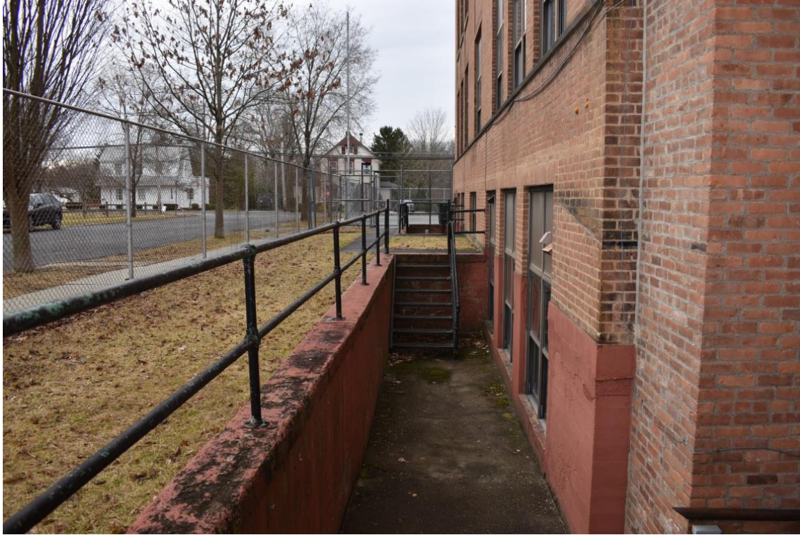
Photo 6: Access points on the eastern side of the building are below grade. View to the south.
