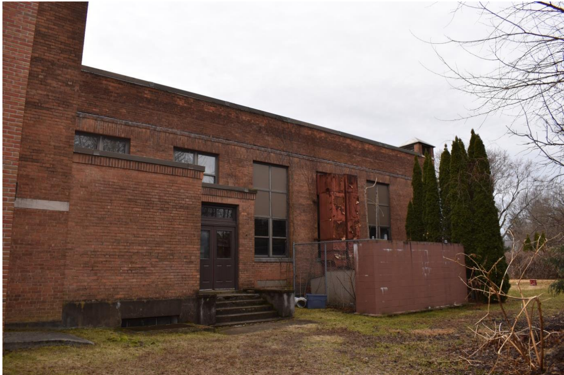
Photo 4: Buried utilities and equipment are located on the northern side of the school building. View to the southwest.
