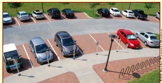
Permeable pavement and brick pavers in the parking lot with reinforced grass overflow parking to the rear.
