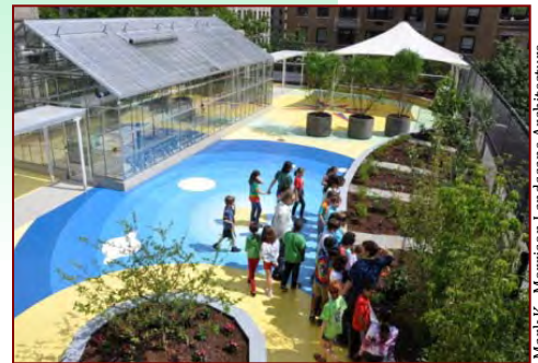
Green roof with greenhouse and vegetable gardens at New York City school reduces runoff and provides students all-season, hands-on ecological education.
