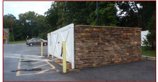
This enclosure features attractive, durable materials that match the adjacent buildings, steel corner posts, separate pedestrian door, and evergreen screening with rear fence.
