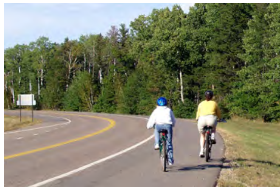
Paved shoulders are most applicable on higher-speed and higher-volume rural roads.
