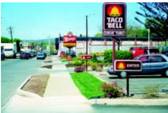
Paired one-way access drives cause multiple curb cuts too close together, lots of traffic conflict points, excessive breaks in the sidewalk, and repetitive enter/exit signs.
