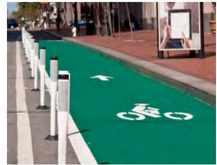
A bike lane can be protected with bollards, planters, or a curb, creating a "cycle track".
