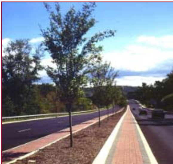
This new section of Route 55 features brick pavers and street trees, which when fully grown will create an attractive boulevard quality and reduce the apparent width of the road.
