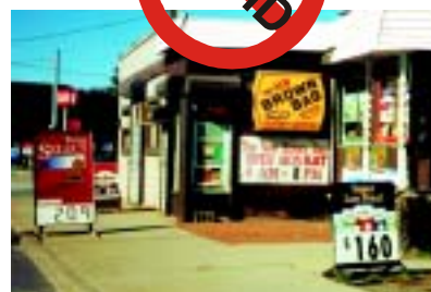
Too many signs, including one blocking the sidewalk, create visual chaos and detract from the entire area.
