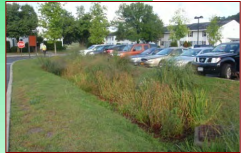
Bioretention swale at Marist College collects runoff from the parking lot, absorbs and filters rainwater, and includes an overflow grate for any flooding.
