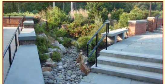
Rain garden built into a planter box at the building entrance.
