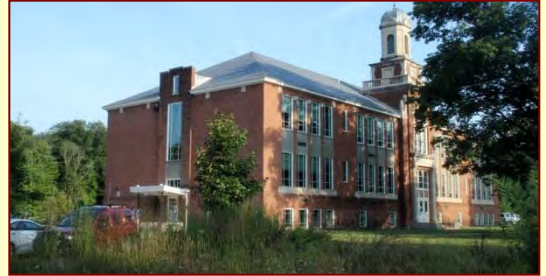
Adaptive reuse of a vacant 1930s school building in the National Landmark Hudson River Historic District.
